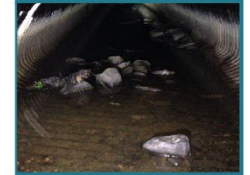
CC00230 CMP Culverted Stream
